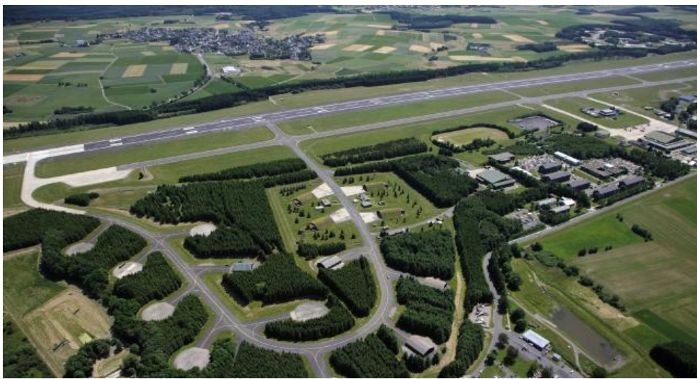
Storage depots at Büchel Air Base in west-central Germany where up to 20 US Air Force B61 thermo-nuclear gravity bombs are stored for use on German Tornado jet fighter/bombers. The base has been the object of nuclear weapons protests for 20 years.
