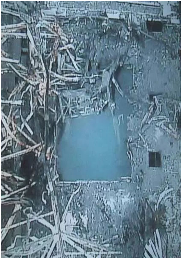
The wrecked waste fuel pool at Japan's Fukushima-Daiichi's reactor No. 3 in March 2013.
