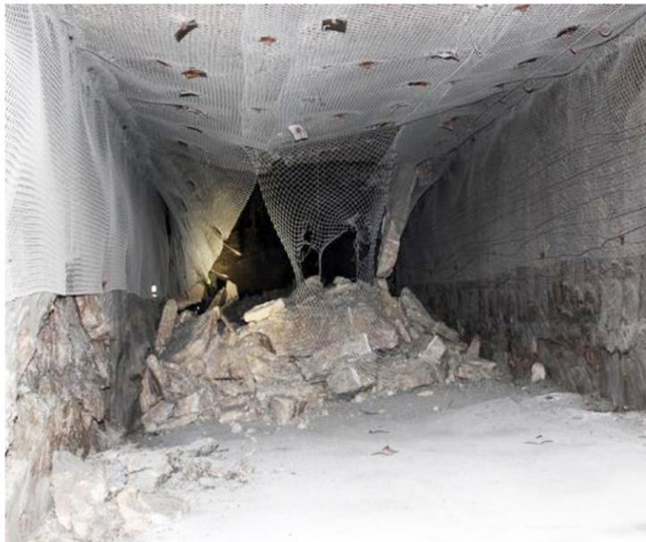
One of two deep-underground tunnel roof collapses that recently caused evacuations of the military radioactive “Waste Isolation Pilot Plant” in New Mexico. Photo: Energy Dept.
