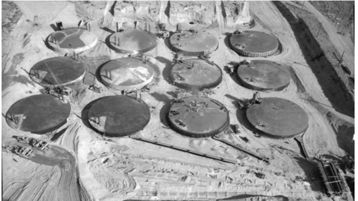
Pictured: Some of the 177 tanks holding 56 million gallons of liquid high-level radioactive wastes at the Hanford Reservation on the Columbia River in Washington state. At least 77 of the tanks are leaking. Over a period of 40 years, nine Hanford reactors along with chemical "reprocessing" to get plutonium for weapons, produced billions of gallons of such waste. At least 450 billion gallons were dumped on land or injected into deep wells. Clean up operations could last 100 years were estimated in 1988 to cost $175 billion. Energy Dept. photo.
