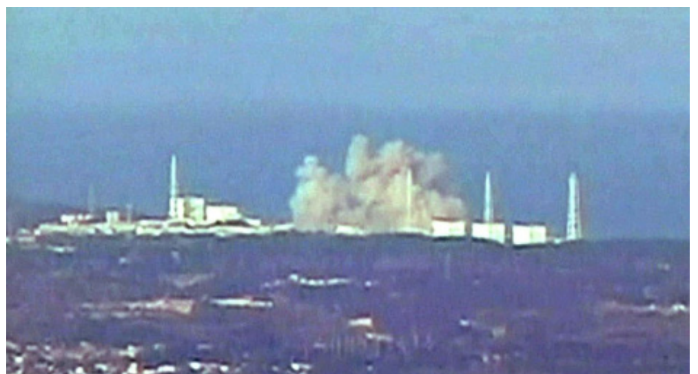
Pictured: One of three large explosions that were a part of Japan's Fukushima-Daiichi radiation disaster that began March 11, 2011 with the country's largest earthquake, the fourth largest since record keeping began in 1900. The quake smashed the reactors' foundations, pipes and off-site electrical supply, causing a "station blackout" that halted water circulation and all cooling of the reactors. A massive tsunami destroyed emergency back-up generators needed for cooling, resulting in meltdowns in three large reactors, enormous radiation releases, and possibly the worst nuclear reactor disaster in history.
