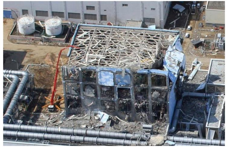
A Reuters image of a Fukushima reactor in ruins following three hydrogen gas explosions that were in turn brought on by meltdowns inside three reactors.
