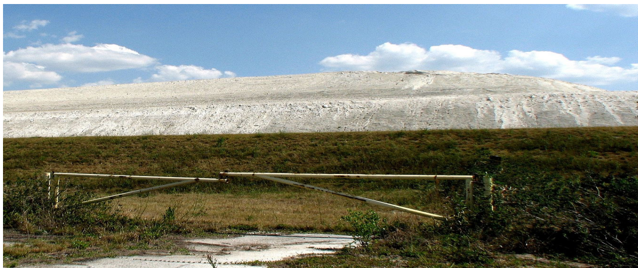
Florida has 25 giant stacks of waste, like this one near Ft. Meade, left by the phosphate fertilizer industry and contaminated with uranium and radon. The mounds can cover 800 acres and be 200 feet high.
