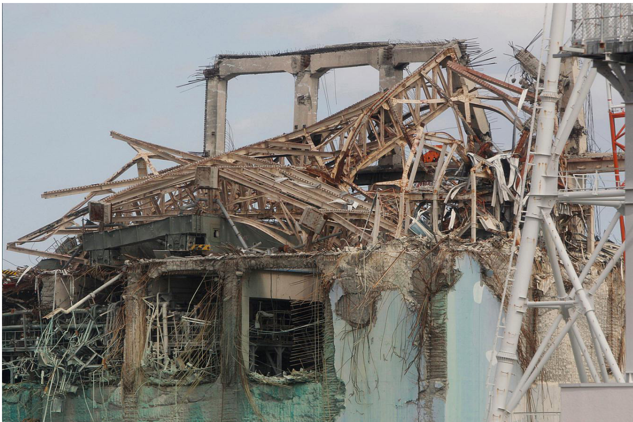
Hydrogen explosions blew apart four of the six reactor containment buildings at Fukushima-Daiichi in March 2011.
