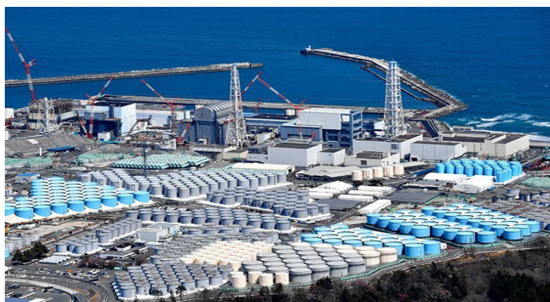
Over 1.3-million tons of wastewater contaminated with dozens of radioactive chemicals left from cooling three reactor core meltdowns stored in tanks at Fukushima Daiichi, in Japan.
