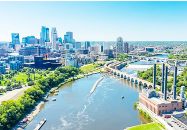
Mississippi River running through Minneapolis, Minn., drinking water for 20 million downstream was contaminated by Monticello reactor leak.
