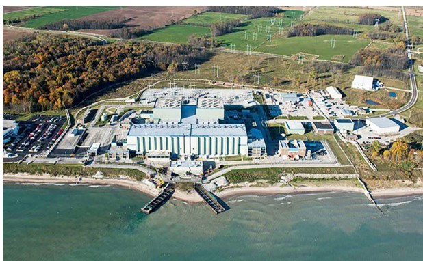
Point Beach Reactor, on Lake Michigan, in Wisconsin. In September, the two reactors on site were awarded license extensions to run until 2050 and 2053. Photo: reddit
